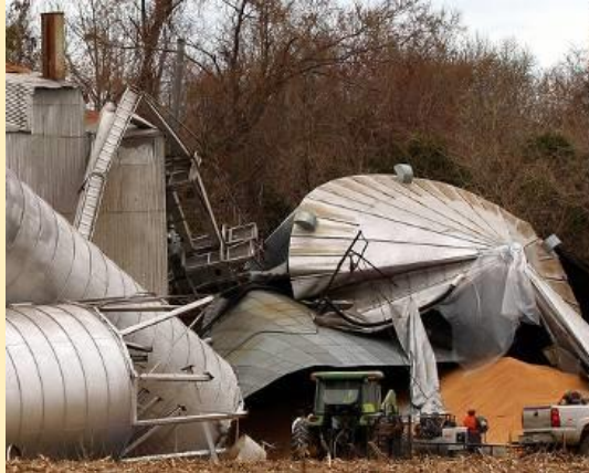
Bridging transfers load to the bin wall
