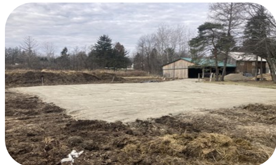
Completed Extended Use Area at Thompson Farm.
