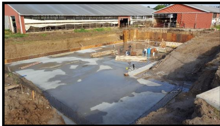
Figure 3 – Footing poured and walls being formed for an ag waste, milkhouse water, and low flow silage leachate collection and storage. Avon (Livingston Co.)
