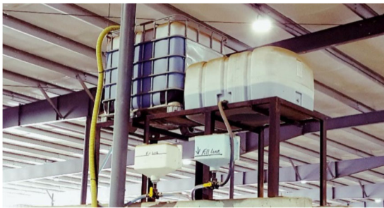
Figure 2 - Elevated totes of premixed footbath solution.
