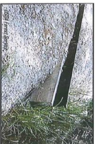
Water deflectors are installed so that 3 inches of rubber belting extends above the surface of the road.
