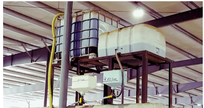
Figure 2 - Elevated totes of premixed footbath solution.
